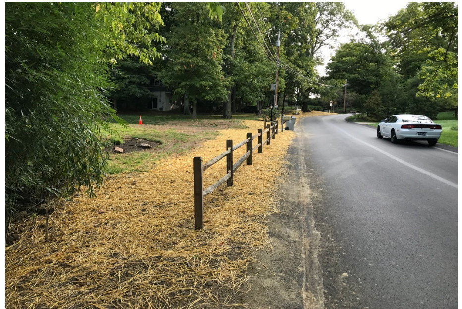
Yard restoration on Robinhood Drive following sewer replacement
