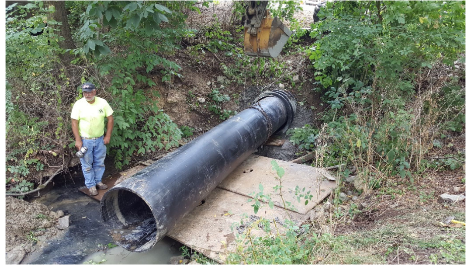
Slip lining operations on Shady Lane
