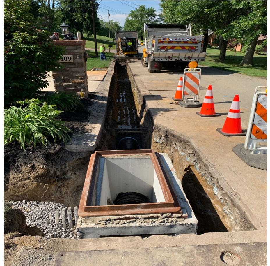
Construction of storm sewer system on Redwood Drive
