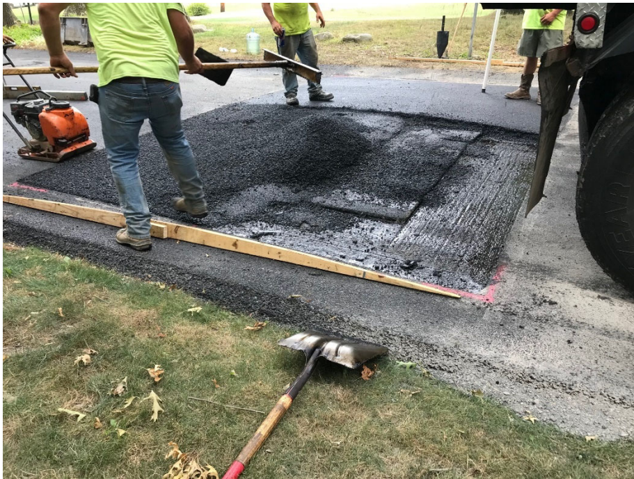
Paving speed hump on Oakwood Road
