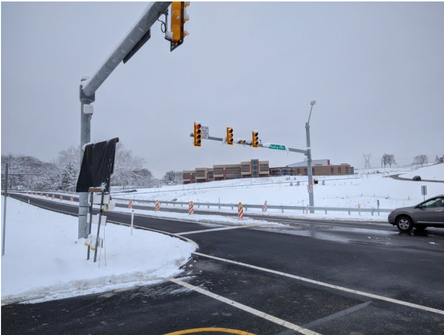
New Traffic signal / intersection of Rolling Hills Drive – Dec. 2020
