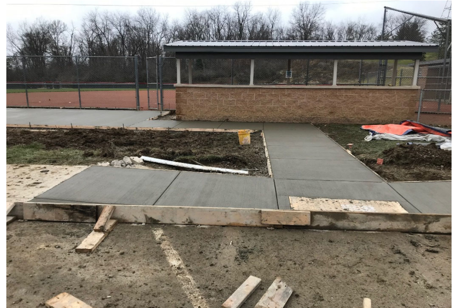
ADA Walkway/Ramp construction at Peterswood Park – Dec. 2020
