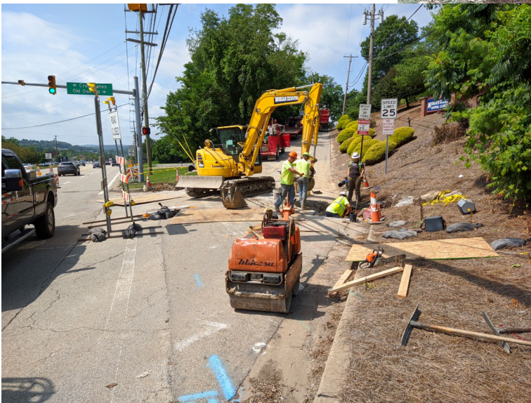
Old Oak storm sewer - July 2021
