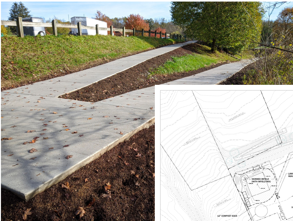
Venetia Park ADA sidewalk
