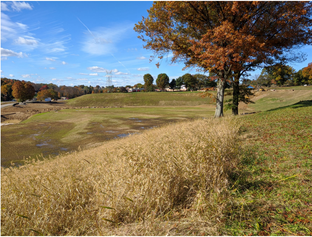
Aquatics Center building pad - November 2021
