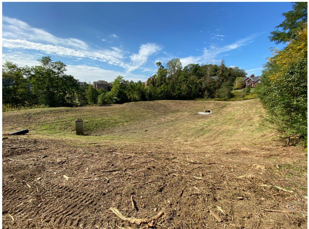
Old Trail 14 SWM Pond - post rehab
