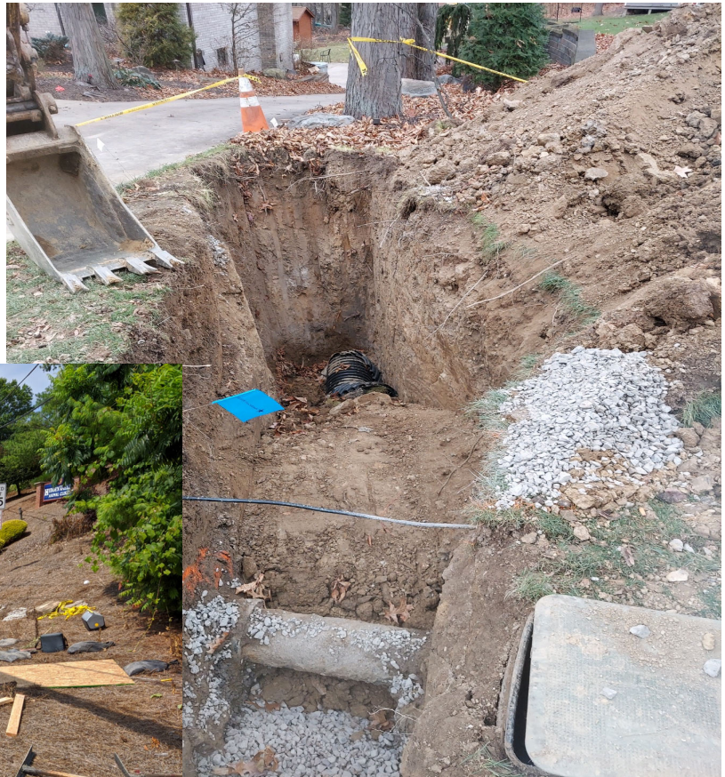
Lintel Drive storm sewer - Nov 2021
