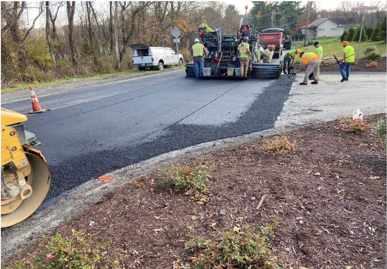
Raised intersection installation - Bower Hill Road
