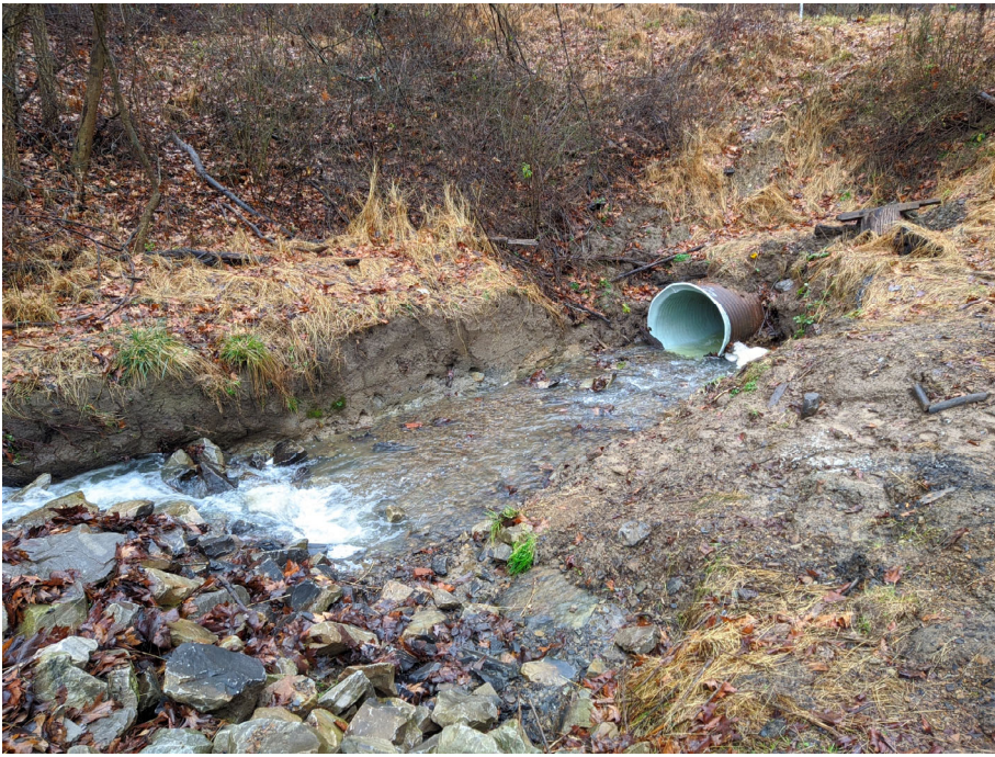
Gateshead culvert - upstream entrance
