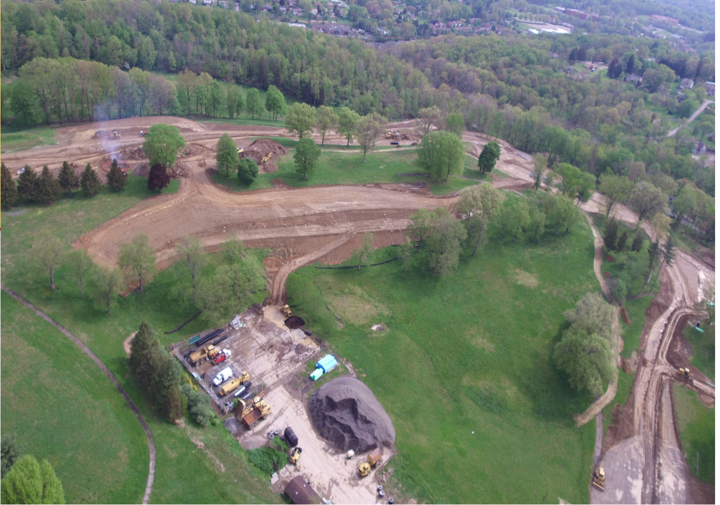
Rolling Hills Park under construction - May 2021
