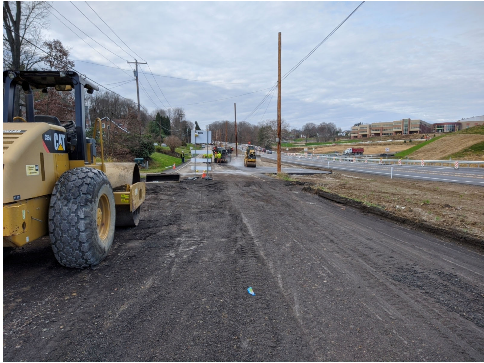
Removal of 'old' East McMurray Road
