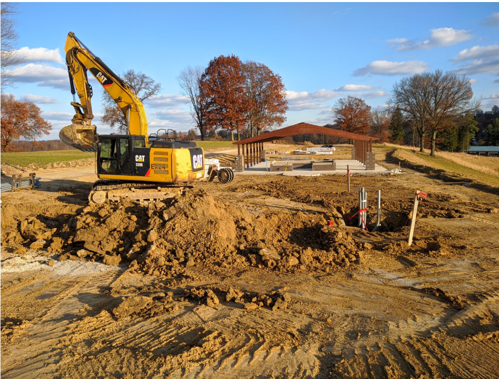
Utility and pavilion construction in Great Lawn area - November 2021
