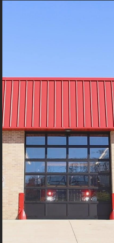
“Garage Door Replacement” video
