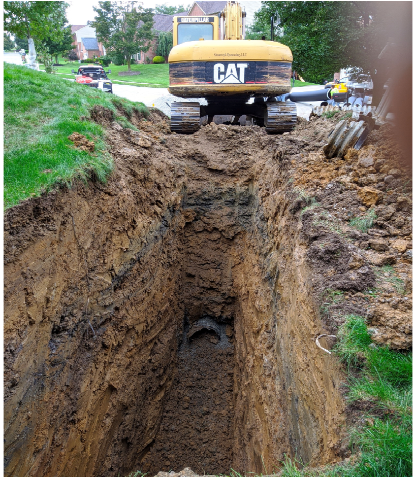
Sand Creek Drive - Emergency storm sewer repair Sept 2022
