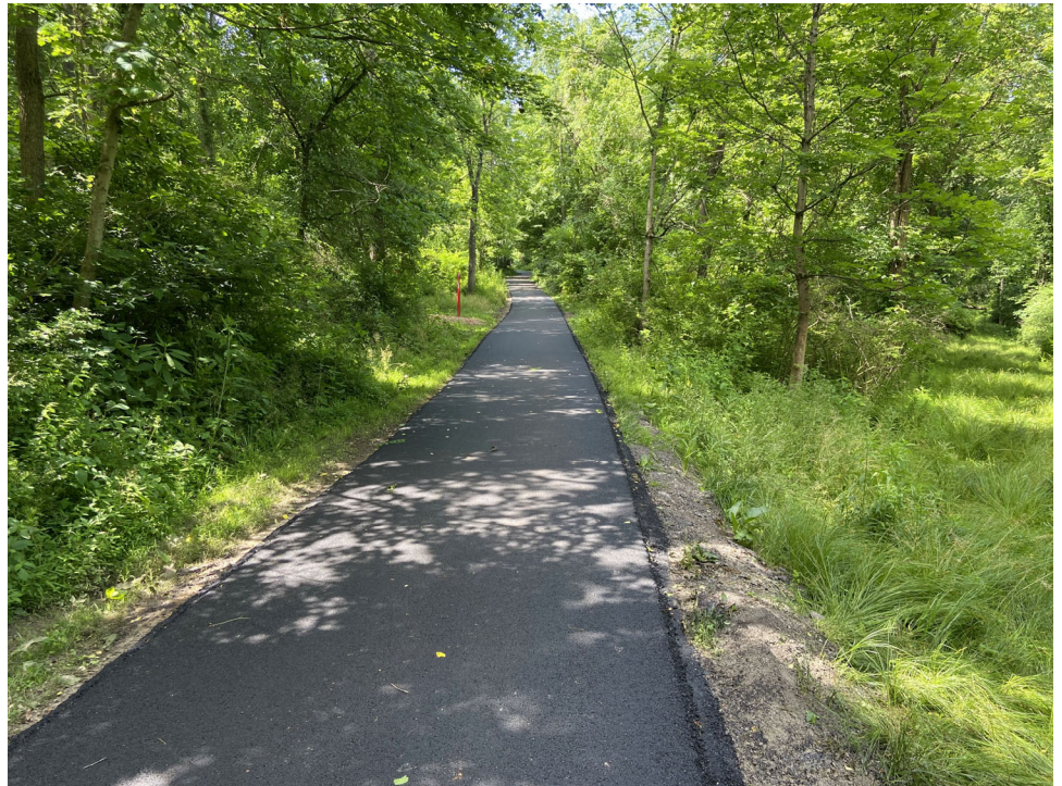
Connector path to Arrowhead Trail - newly paved June 2022
