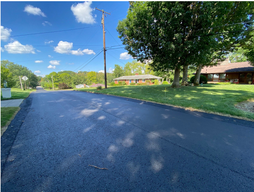
Rutledge Drive following completion of binder course - August 2022
