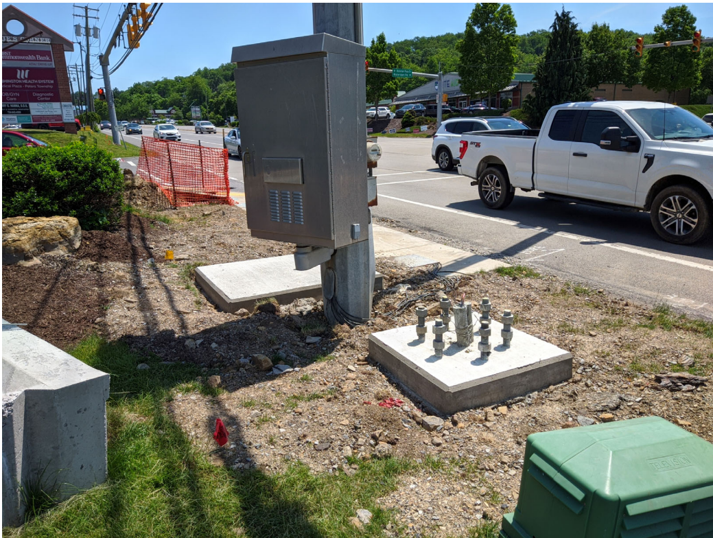
Waterdam Traffic Signal repairs
