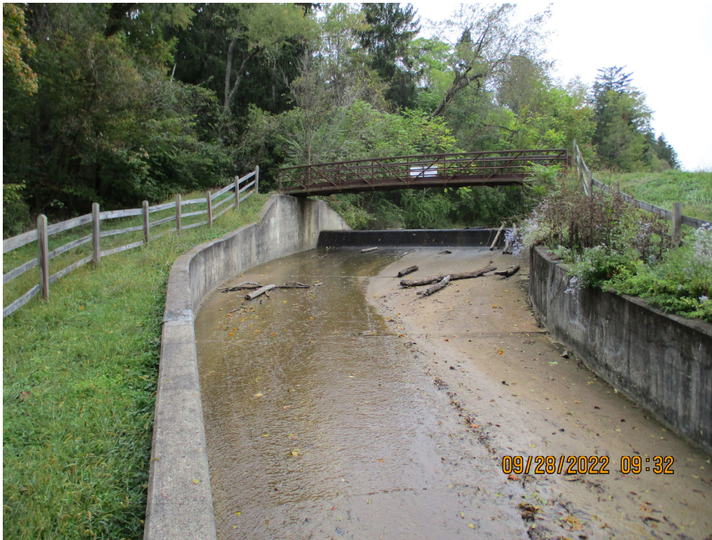
Peters Lake Spillway - Sept 2022
