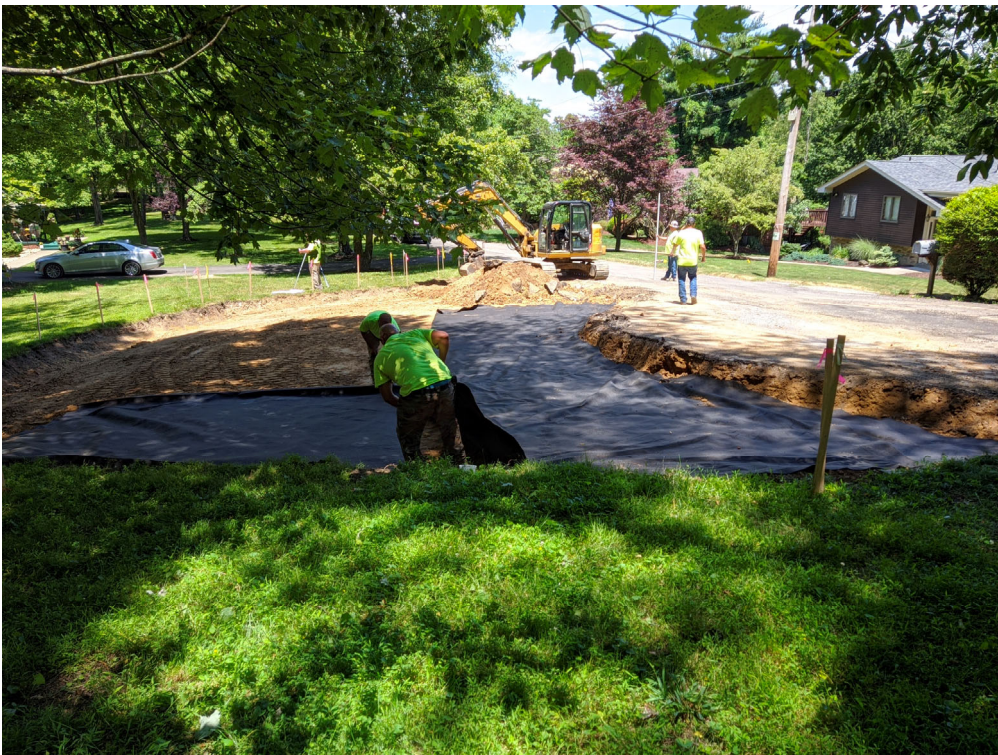
Construction of new cul-de-sac - July 2022
