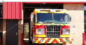
Fire Station #1 Garage Door Replacement 477 views
