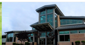
CRC Renovations 813 views
