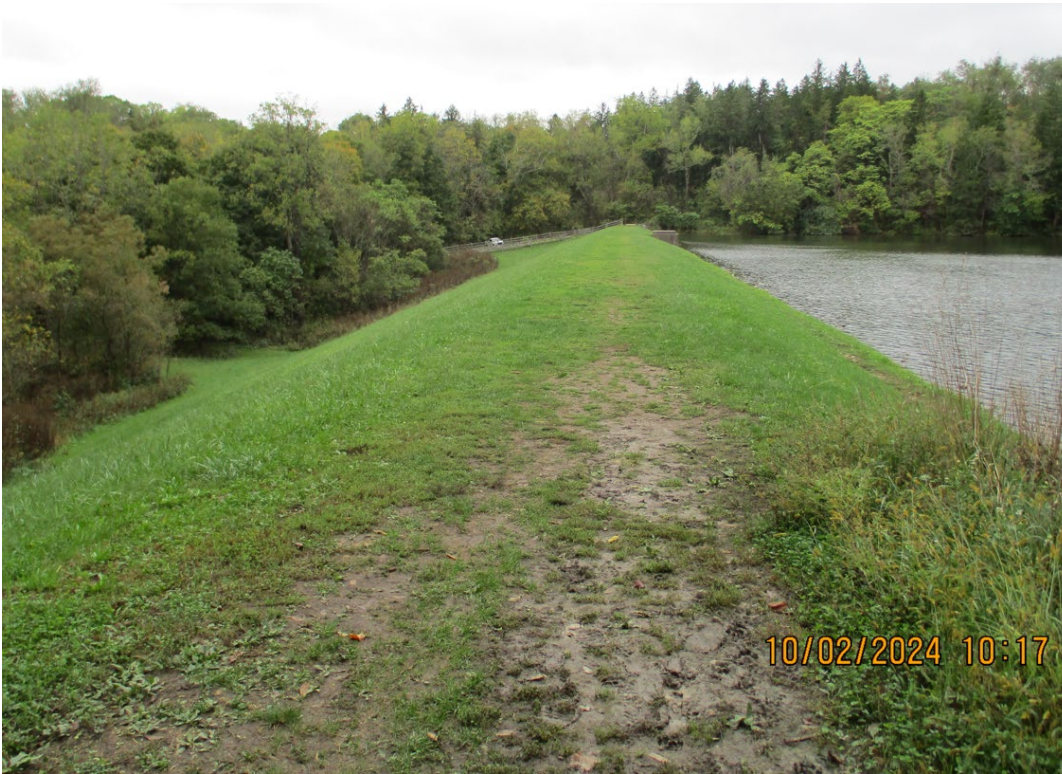
Peters Lake Embankment - Oct 2024
