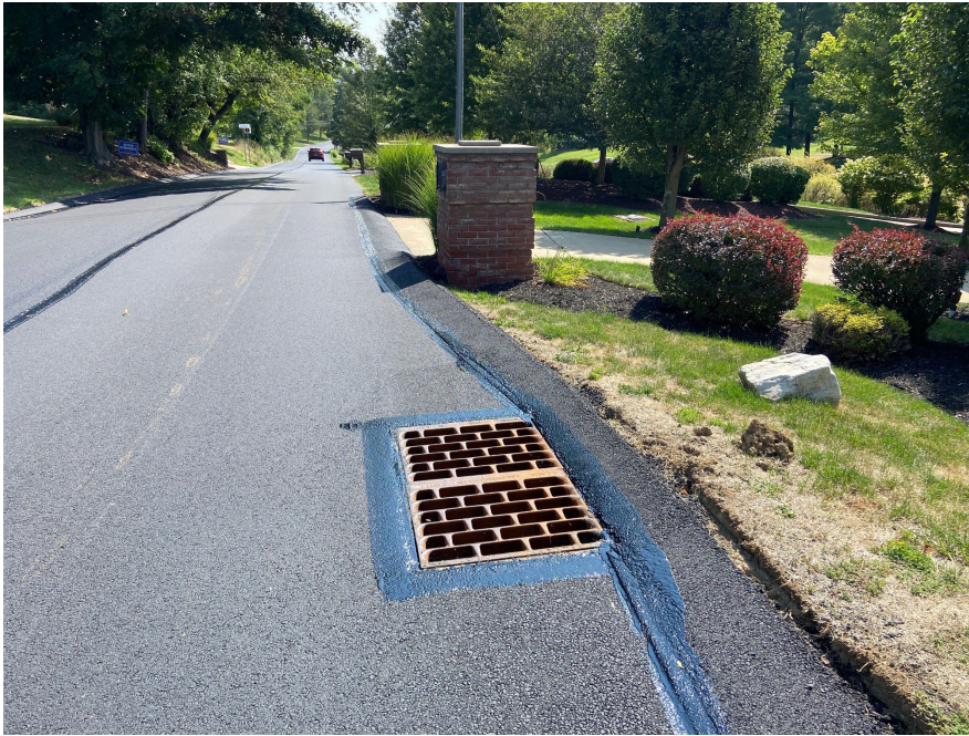
Finished wearing course - Springdale Road
