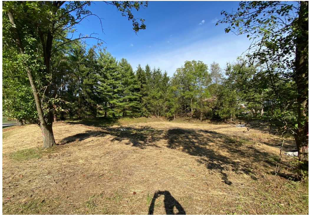
Ross Creek SWM Facility - rehab in progress Sept 2024
