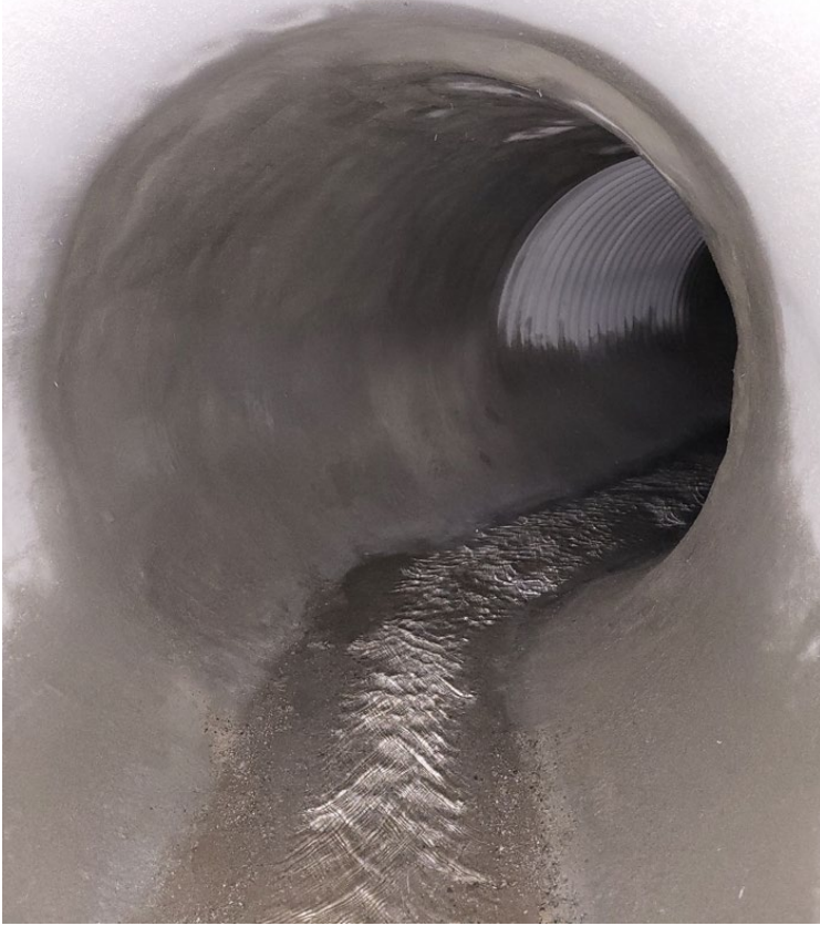
Camp Lane culvert - finished lining - February 2024
