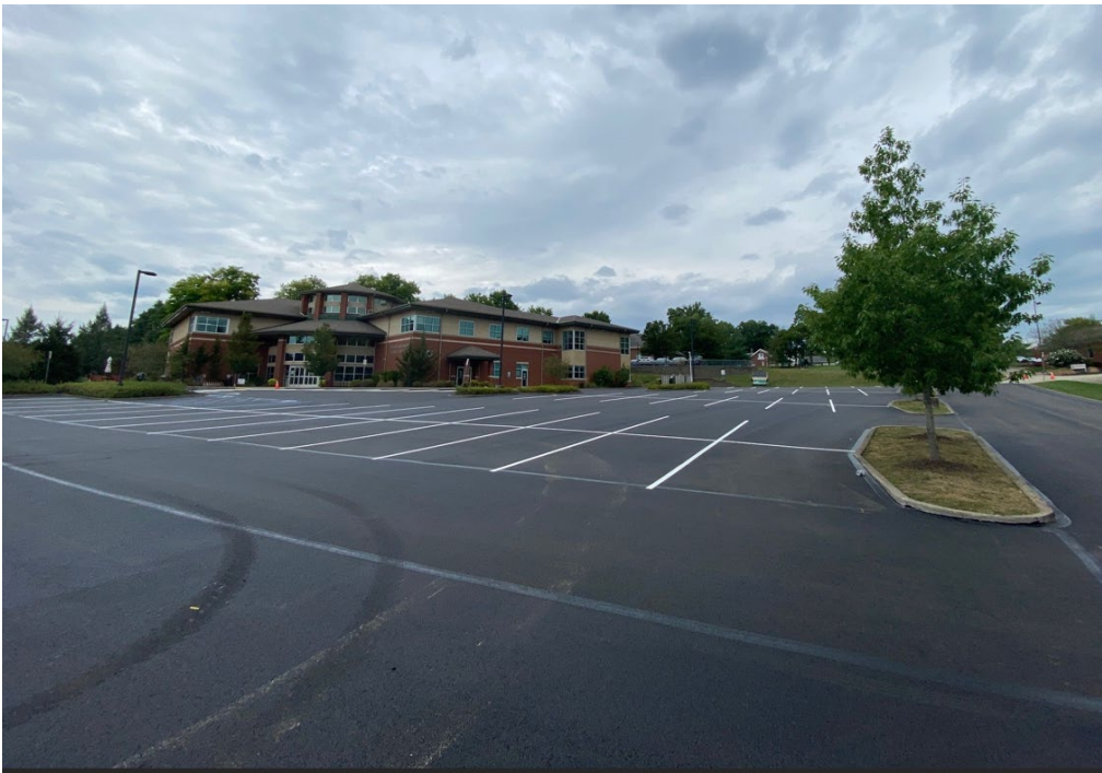
Finished pavement and markings at the Municipal Complex – August 2024
