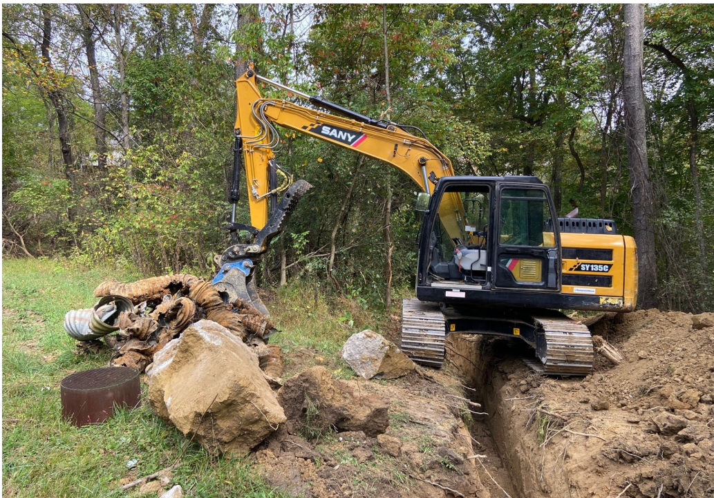
Colony Manor detention pond (north) - demolition/removal of CMP outlet pipe
