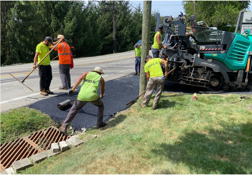
Paving at the bottom of Brookdale Road - July 2025
