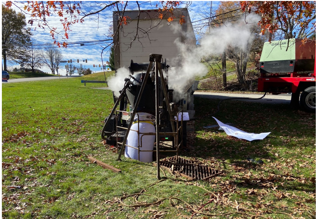
Center Church Road cured-in-place lining - November 2025
