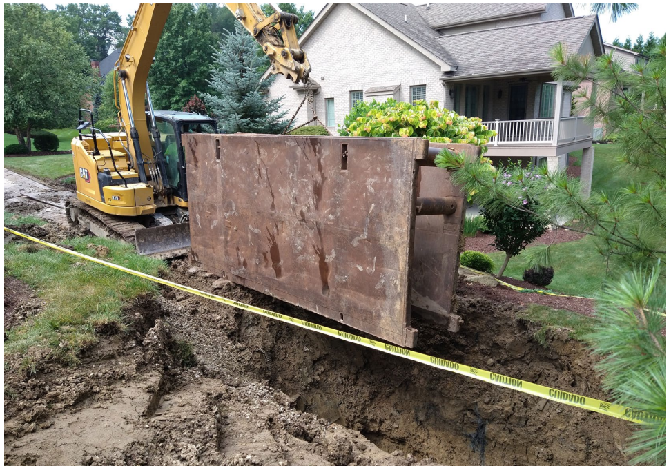
Sussex Way emergency repair - July 2025
